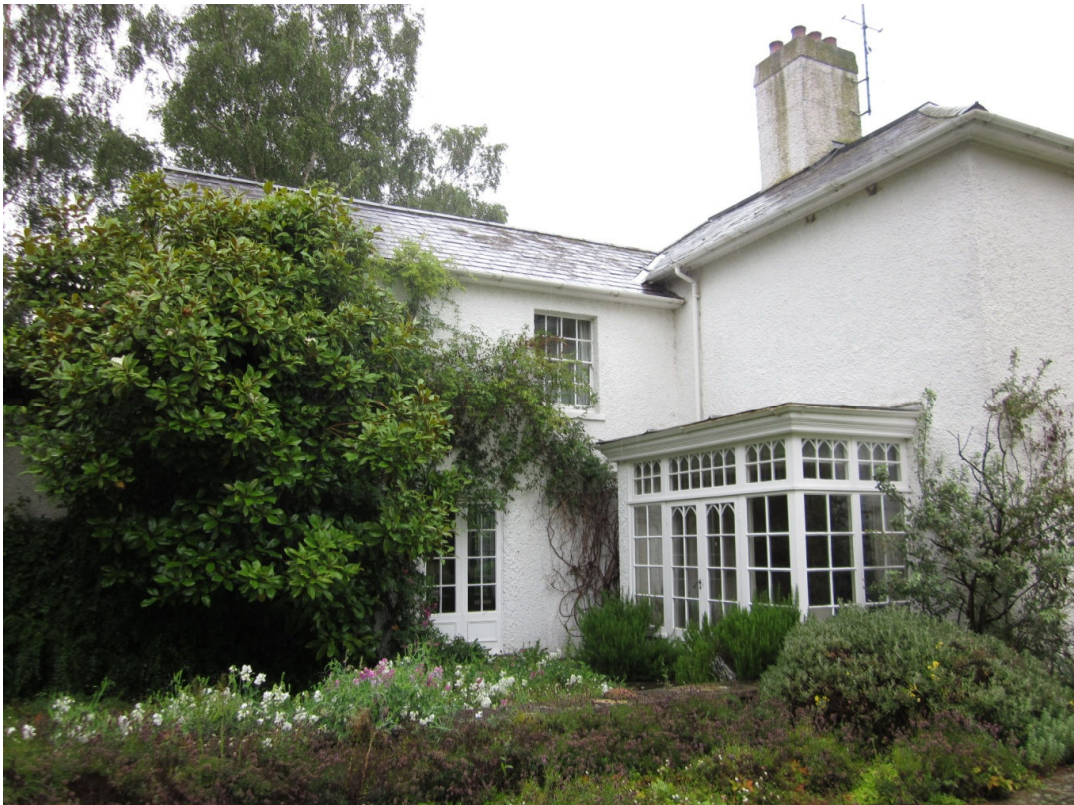
South west elevation, main house and service (west) wing
