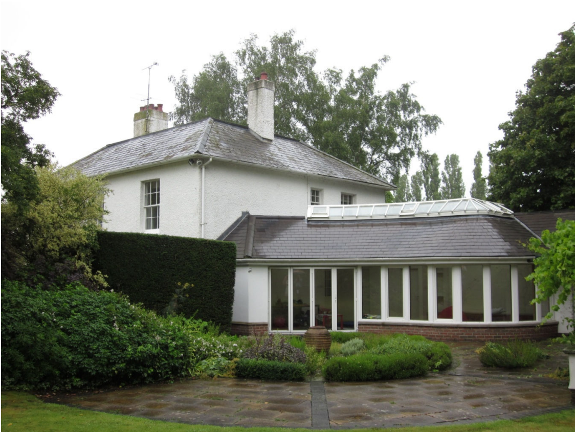
South east elevation, main house and conservatory
